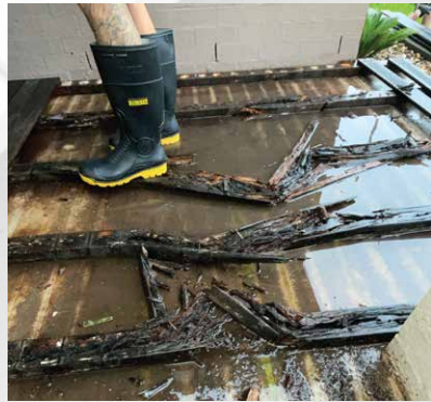
2 year old H3 deck frame on concrete
